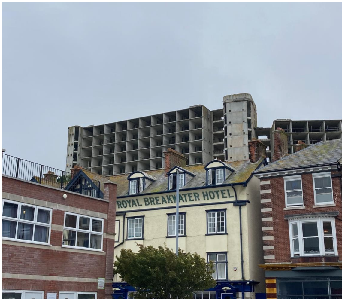
Figure 3: The Royal Breakwater Hotel is towered over by a derelict block, which once served as barracks for the Royal Navy. Work on this building was abandoned, leaving it in its current state of dilapidation.
