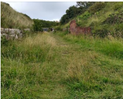
Footpath to High Angle Battery - widening
